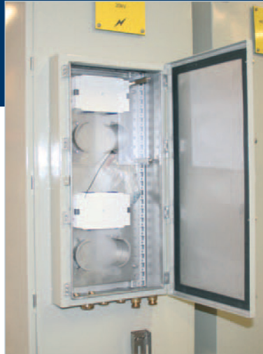
Cabinet for Optical Fiber Termination (Ex op is) integrated in High Voltage cabinet
