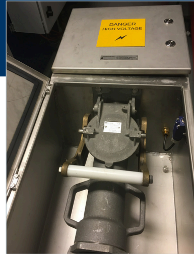
3-Phase 11kV Plugable solution, Max 3x240mm 2
