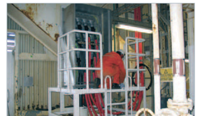
Installation on site
